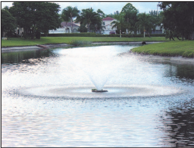
Fig 36.11 | Water aerator for a large pond.
