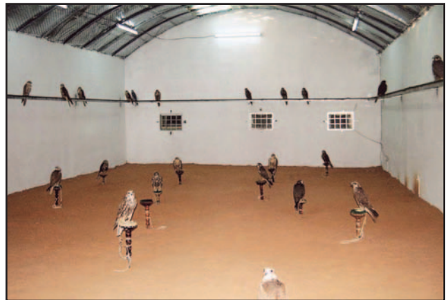
Fig 40.5 | A typical free-flying molting room in the Middle East measures 15 x 8 x 5 m and is provided with red desert sand as a substrate. A single platform-type perch is placed around the room. Some birds have already been released, while others wait on stands until they are settled into the new environment.
